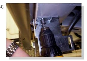
Attach FL230 at 19, (20) 32, 50 and 67 inch locations with 5/16" bolt and nut and two 3/4" long self drilling screws. Pre drill hole for self taping screw with 1/8" drill bit.
