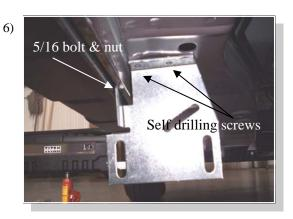
Attach FL141 at 43" and 59" locations with one 5/16" bolt and nuts and two self drilling screws.
