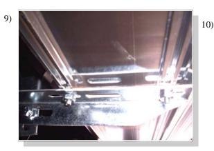
Place the board on the brackets with the bolts through the slots. Fasten with 1/4" flanged nuts.
