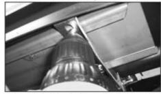
8. For Molded Boards: Position board where you want it. Install self-tapping bolts through bracket into the shoulder of steel channel on bottom of board.
