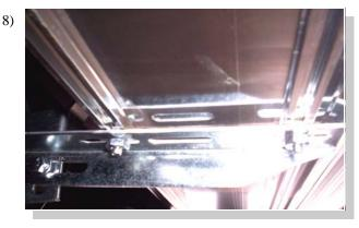
Place the board on the brackets with the bolts through the slots. Fasten with 1/4" nuts.
