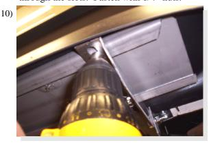
For Molded Boards: Position board where you want it. Install self tapping bolts through bracket into the shoulder of the steel channel on the bottom of the board.
