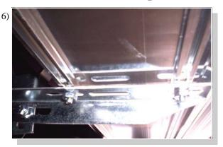
Place the board on the brackets with the bolts through the slots. Fasten with 1/4" nuts.
