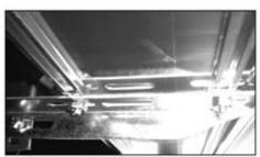
6.Place 1/4" bolts through bracket step support and secure board with 1/4" hex nuts.
