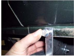
At 4.5" measurement install FL200 by inserting 5/16" flanged bolt through hole in bracket and pinch weld, and attach with 5/16" flanged nut. Snug but don't tighten.
