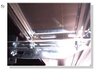
Insert one square head bolt into each track for each bracket. Set board on brackets with 1/4" bolts going through slots on bracket, attach with the 1/4" nuts. Level board and tighten down any and all loose nuts and bolts. Repeat for the other side.
