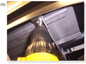
Position board where you want it. Install self taping bolts through bracket into the shoulder of the steel channel on the bottom of the board.
