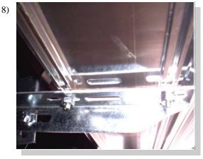
Place the board on the brackets with the bolts through the slots. Fasten with 1/4" nuts.
