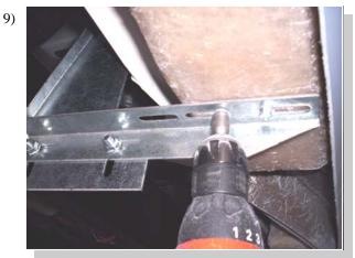
Using self drilling screws attach the board to the angle brackets making sure you are drilling into steel mounting pad. Level board and tighten any remaining loose bolts at this time.
