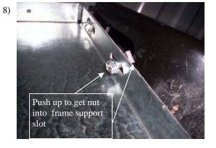
Once the FL172 is pushed up you'll need to push the lower bolt up in the slot and turn the reinforcement nut to fit into large slot in frame support. Make sure reinforcement nut is catching frame support, straighten and push up bracket then snug lower bolt.
