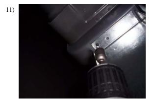
At the top of the bracket you will see 2 holes, straighten bracket and install 2 self drilling screws.
