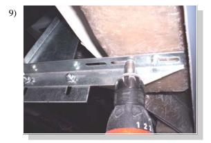
Using self drilling screws attach the board to the angle brackets. Level board and tighten any remaining loose bolts at this time.
