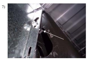
Take FL172 with nut attached as in step 6, and insert the large keyhole slot over the bolt head **FIG** # **5**, angling the FL172 to allow access to rear of bolt through large frame support slot. You will need to reach through large slot and hold the bolt from falling into frame support. Push up on bracket when head is through key hole slot.
