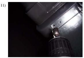
At the top of the bracket you will see 2 holes, straighten bracket and install 2 self drilling screws.
