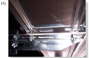
Place the board on the brackets with the bolts through the slots. Fasten with 1/4" nuts. Straighten and level board, tighten bolts and nuts.
