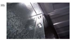
Bracket should look like this when installed correctly
