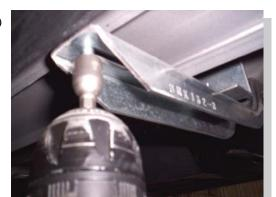
Place the board on the brackets. Attach with #14 self drilling screws. You may need to adjust channels for level and Straightness.
