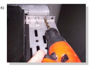
Attach FL73 to support with 5/16" bolt and nut. You will need to drill a 5/16" hole through the support for the second bolt.
