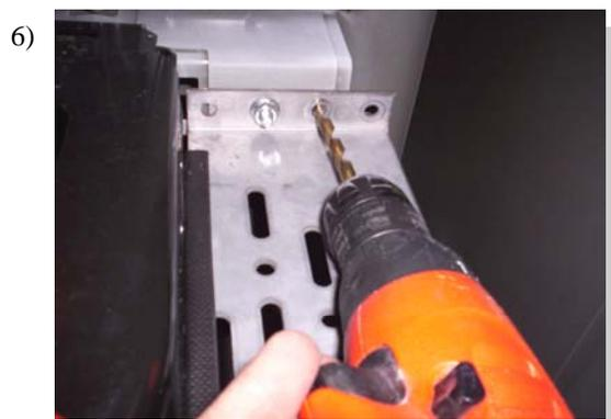
Attach FL73 to support with 5/16" bolt and nut. You will need to drill a 5/16" hole through the support for the second bolt.
