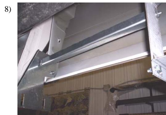
Attach CH07 brace between the two brackets with 5/16" bolts and nuts.
