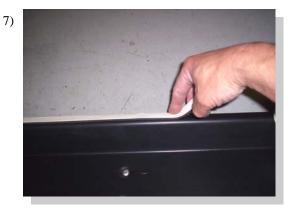
Apply foam tape to top edge of the board.
