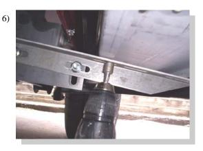
Place the board on the brackets. Attach with 3/4" long self drilling screws. Level board and tighten all bolts.
