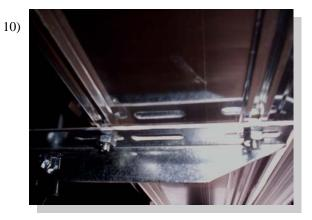
Place the board on brackets with bolts through slots. Attach with 1/4" nuts.
