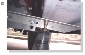
For plastic boards, place board on brackets to desired location. Attach by using 3/4" long self drilling screw into the steel support under the board.
