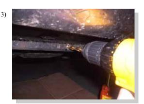
Using a 23/64" drill bit, drill a hole through the pinch weld at marks made in step two.
