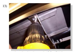
Fasten board to brackets with 3/4" self drilling screws.
