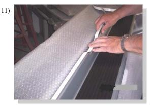
Apply foam tape to rear lip of board and apply the step tread.
