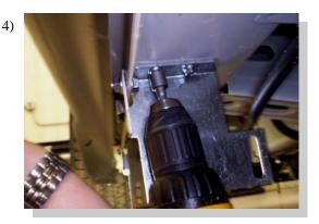
Attach FL129 at 19, (20) 32, 50 and 67 inch locations with 5/16" bolt and nut and two 3/4" long self drilling screws. Pre drill hole for self taping screw with 1/8" drill bit.
